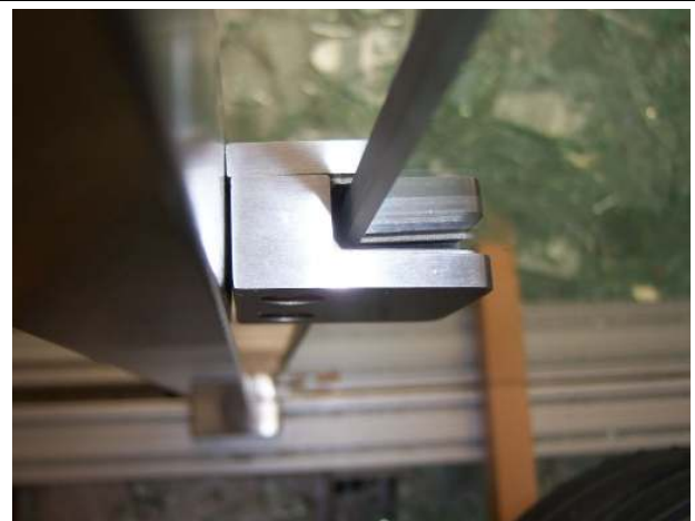
Fig. 16: detail, fixed glass pane in glass clamp model „SQUARE“
